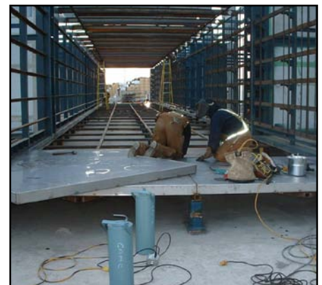
A 4" stainless steel floor is installed in a new WESTMILL™ 6-deck dryer.
