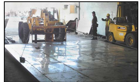
A stainless steel floor module is pushed into a dryer from the end.
